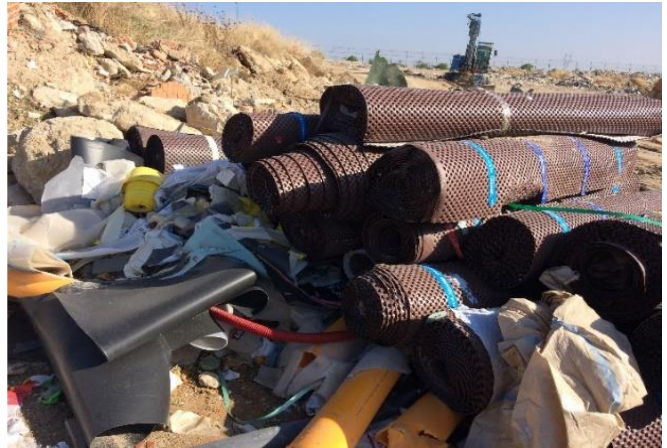
Fig.1 Residues stored in the Complex Treatment of Construction and Demolition Waste located in El Molar, Madrid, Spain.
