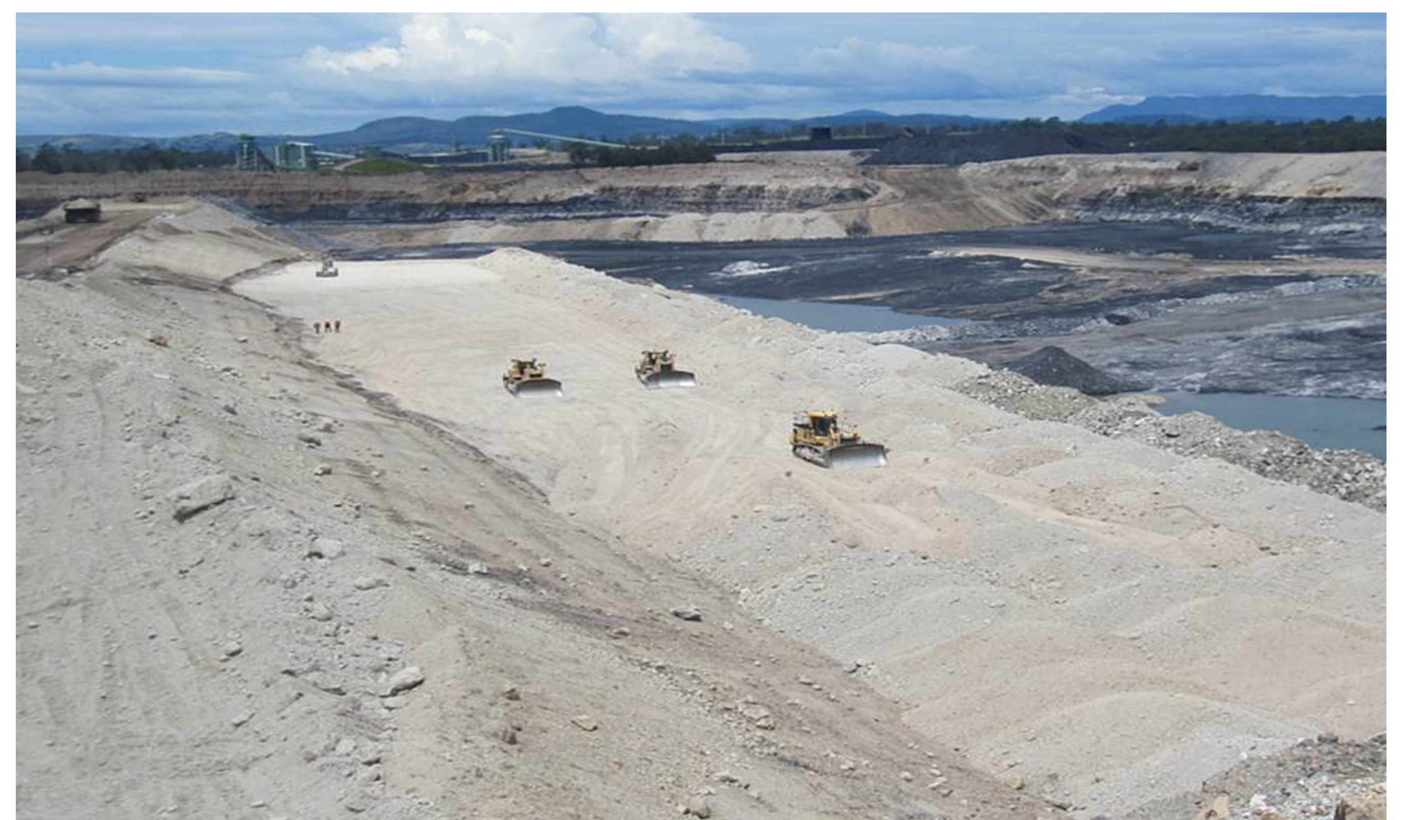
Figure 3: Dozers working on a tailings dam (kce.com.au)
