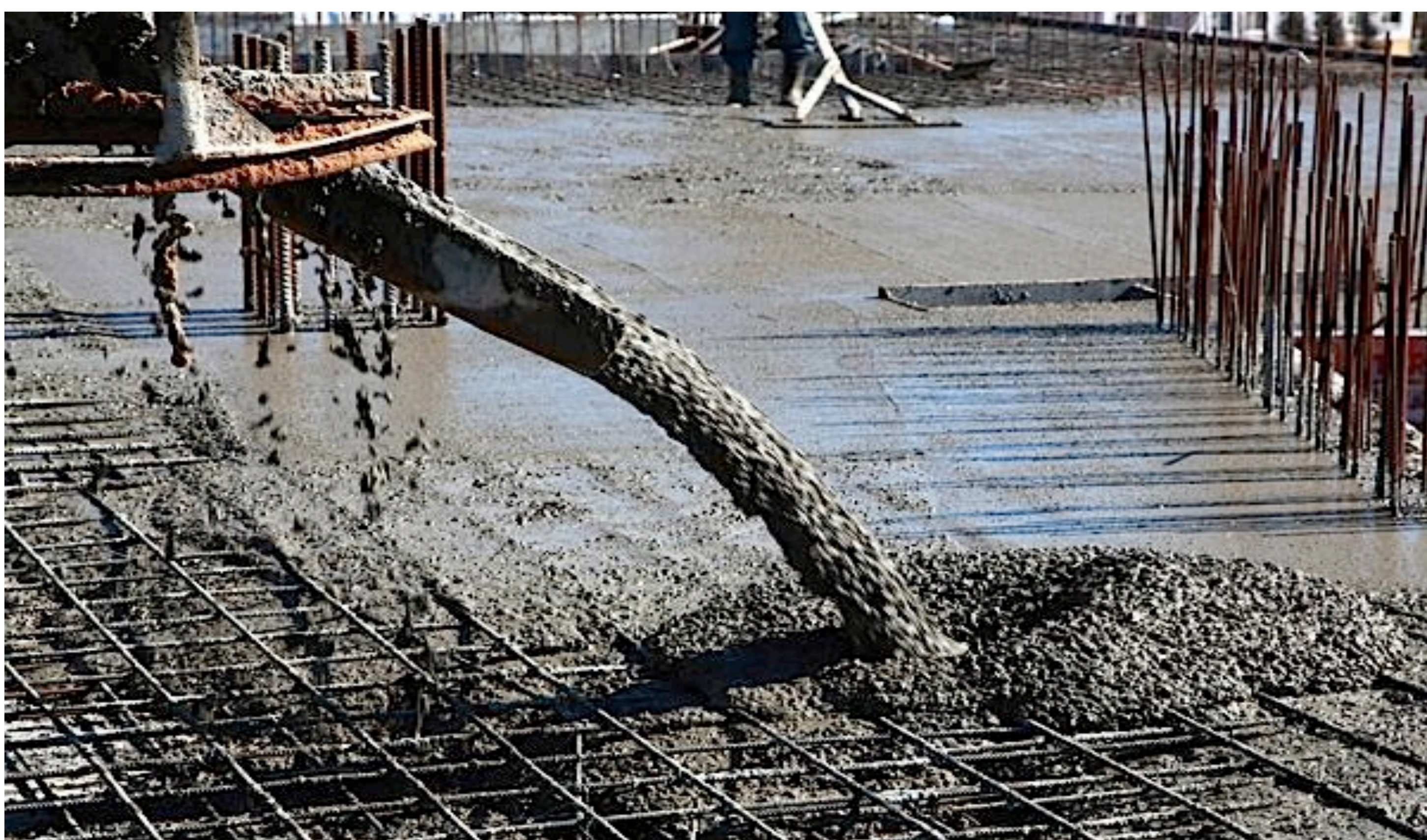
Figure 2: Concrete being used at construction site (declara.com)
