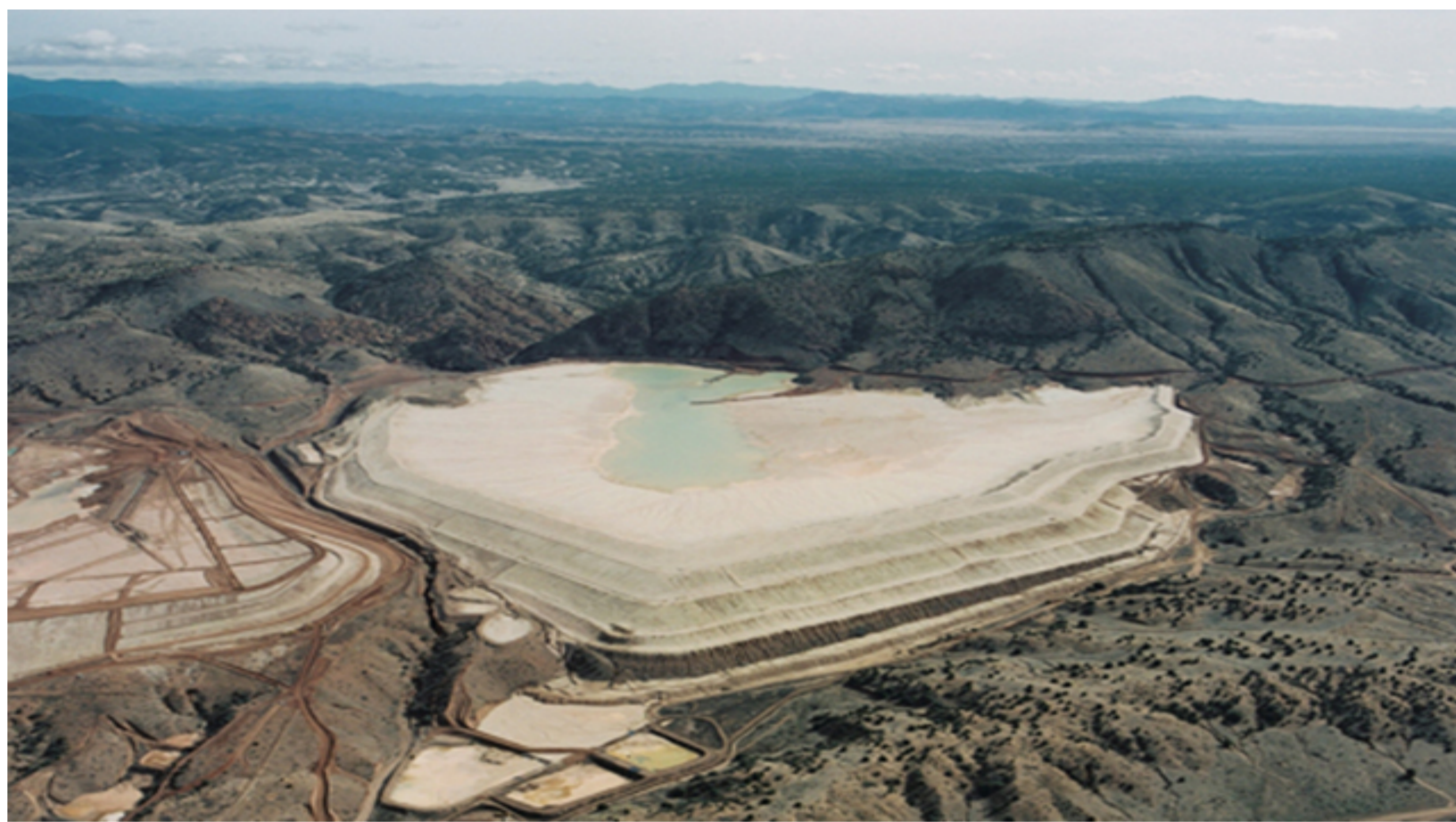
Figure 1: Tyrone Mine's Tailings dam, New Mexico (m3eng.com)
